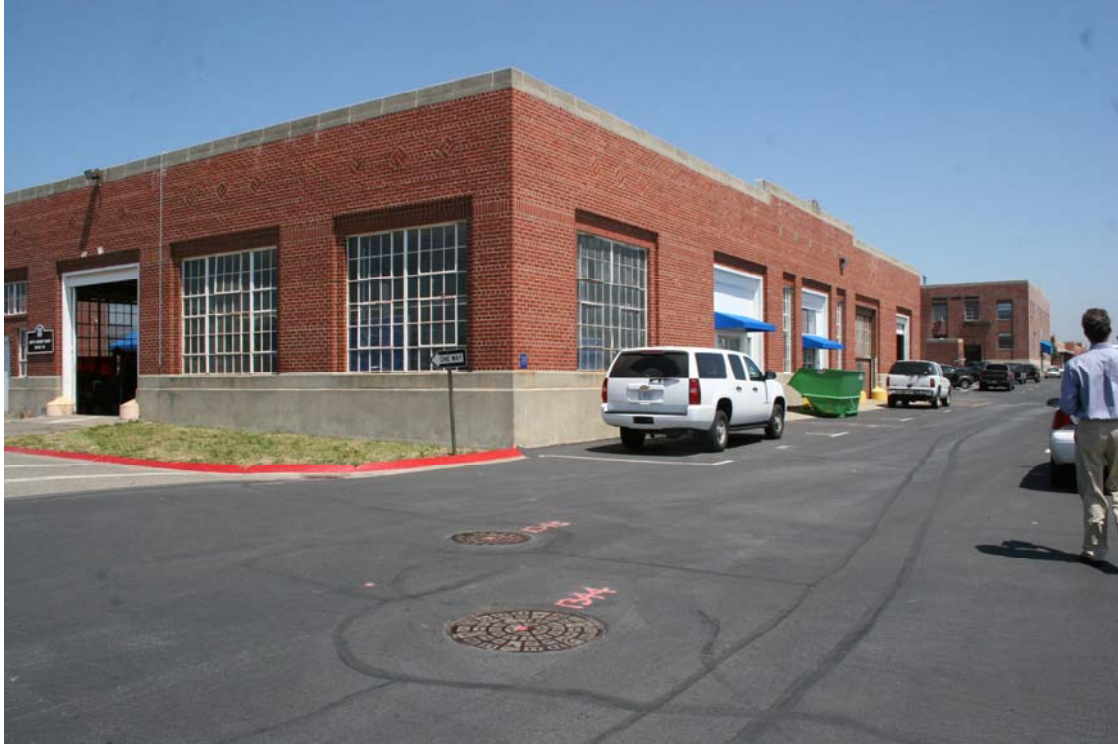
Figure 7: Adjacent building at North-east corner of Spencer Road and Icarus Drive
