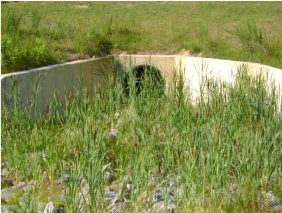
Photo #4: Image of headwall at upstream end of outfall pipe.
