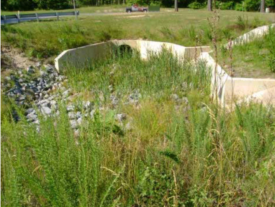
Photo #5: Rip-rap lined basin at upstream end of outfall pipe.
